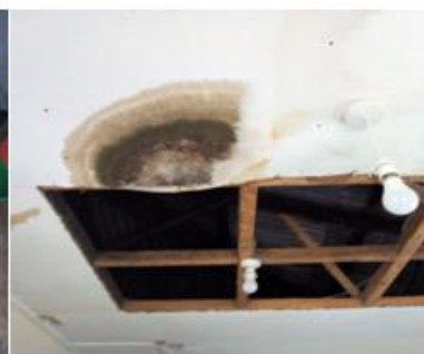
2Ceiling of facility at Nyabani HCIII
