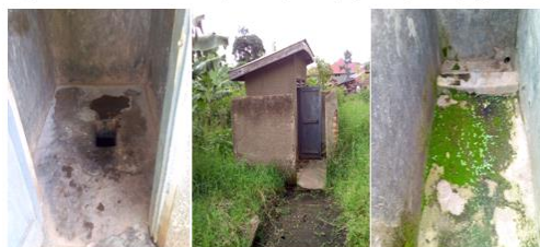
Sanitation status at Kasenda HCIII in Kabarole district
